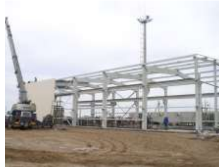
Industrial pump station field Kumkol, Karagandinskaya oblast 15x30x6,35 m. Steel structures weight 30 t
