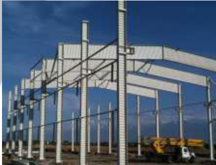
Plant for the production of sanitary paper, RK, Almaty, Steel structures weight 435 t
