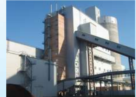
Cement plant, Novotroitsk (group of buildings). Steel structures weight 5 262 t
