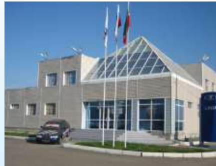
Autocenter, Kazan 18,82x24x4,72 m Steel structures weight 30 t
