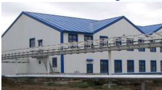
Steel structures of buildings for piping of the objects «Eastern Siberia - Pacific Ocean», Station Lena. Steel structures weight 1900 t
