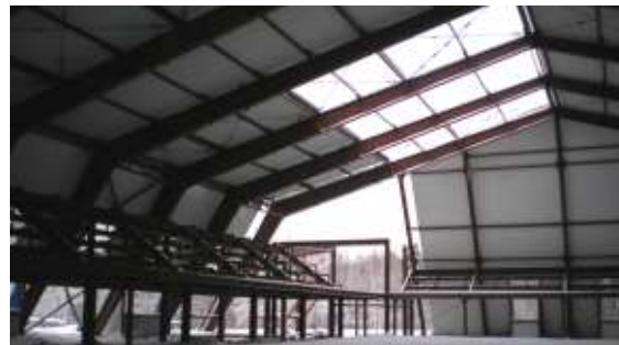
Sports and recreation centre, Zarechniy 50x60x8,1 + 35x45x7,5 + 15x15x15. Steel structures weight 300 t
