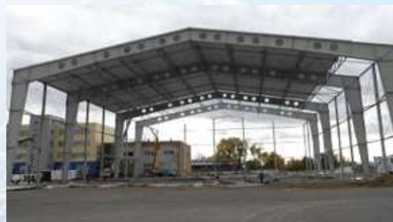
Airshed, Orenburg 51x75x15 m. Steel structures weight 313 t
