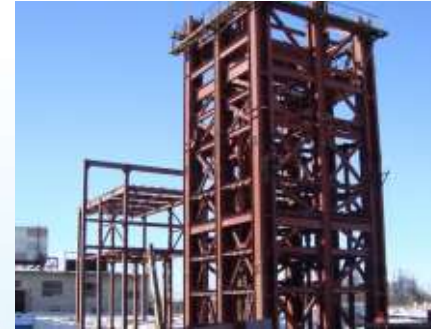
Headgear complex of the mine «Novaya». Puppet head and pithead building, Gay. Steel structures weight 2 588 t
