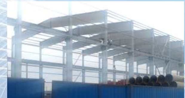
Concrete goods, Atyrau, RK 24+19x140 m. Steel structures weight 265 t
