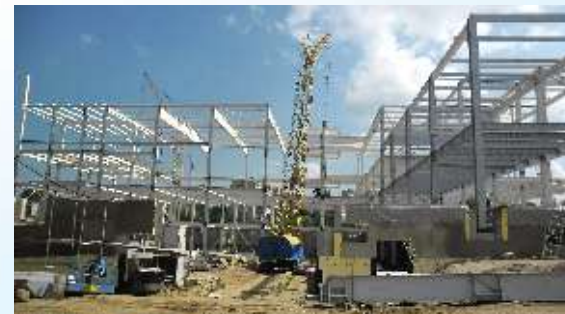
Sport complex with swimming pool, Khabarovsk 68x66,375x9,340/14,500 m. Steel structures weight 650 t
