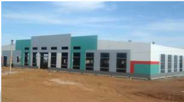
Plant shell for fiber glass, Elabuga (group of buildings). Steel structures weight 3000 t
