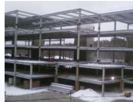
Exhibition complex «Crocus Expo», Moscow. Steel structures weight 730 t
