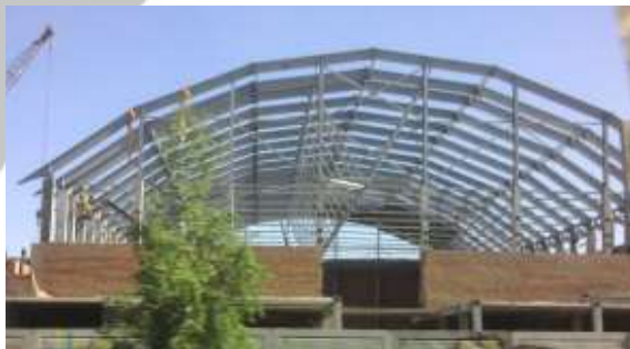
Ice palace, Novotroitsk 75x43x21, 462 m. Steel structures weight 278, 896 t
