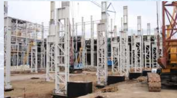
Steel structures for the plant, Kamensk Uralsk. Steel structures weight 1956 t
